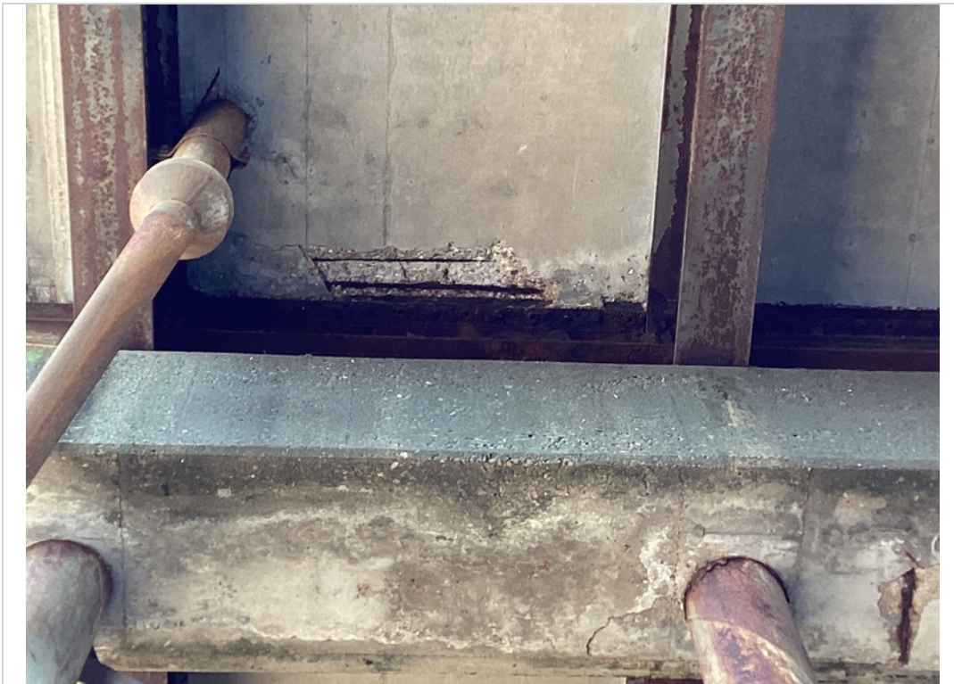
Rebar spall - bay C, span 2, near Bent #1
