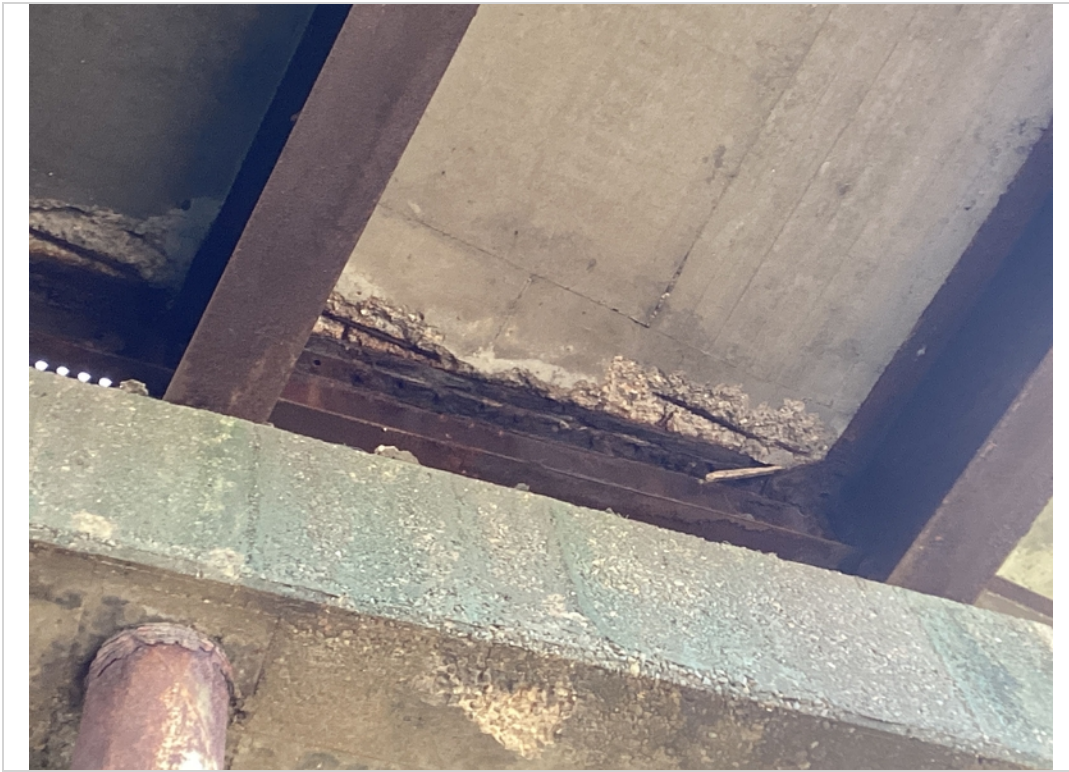
Span 16, bent 16, bay C - rebar spalls
