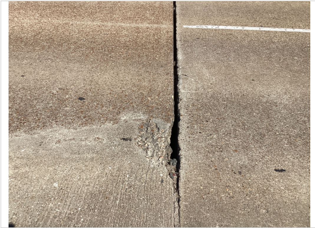
Start of span 8 - joint missing filler, spalling, hole through
