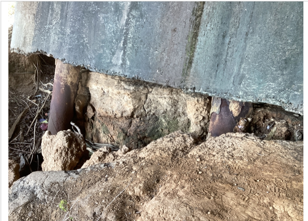
Erosion, exposed piles at abutment 1
