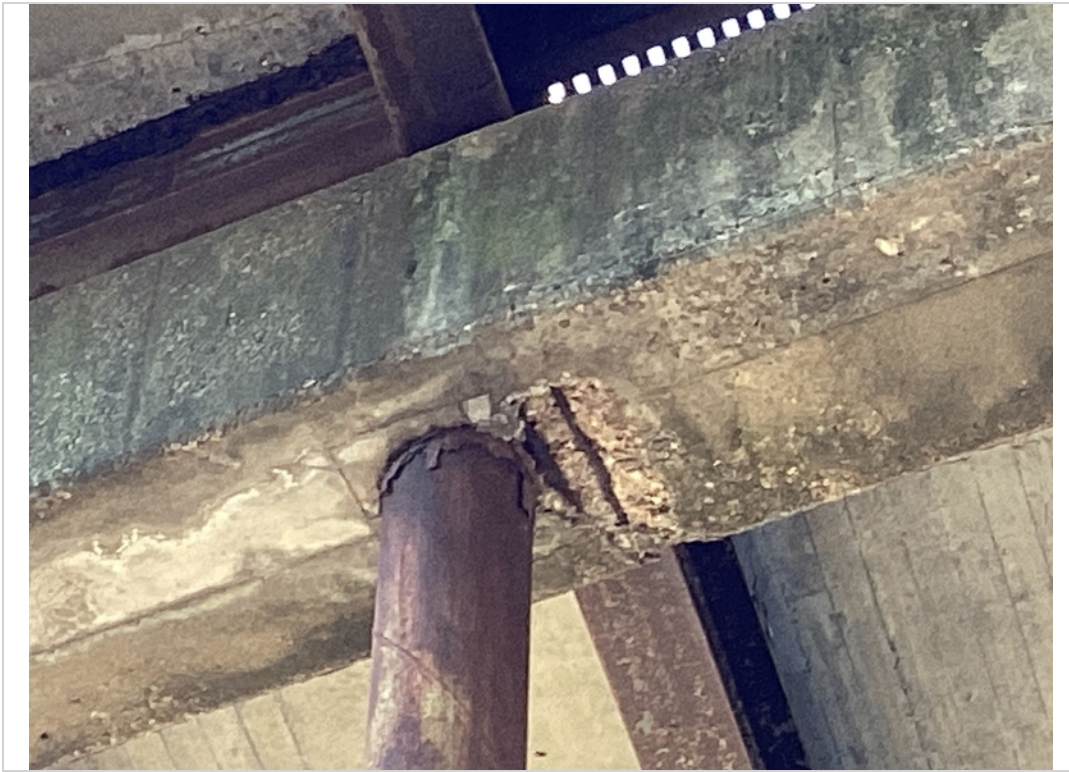
Rebar spall, rust, corrosion - bent 9, column C, looking back
