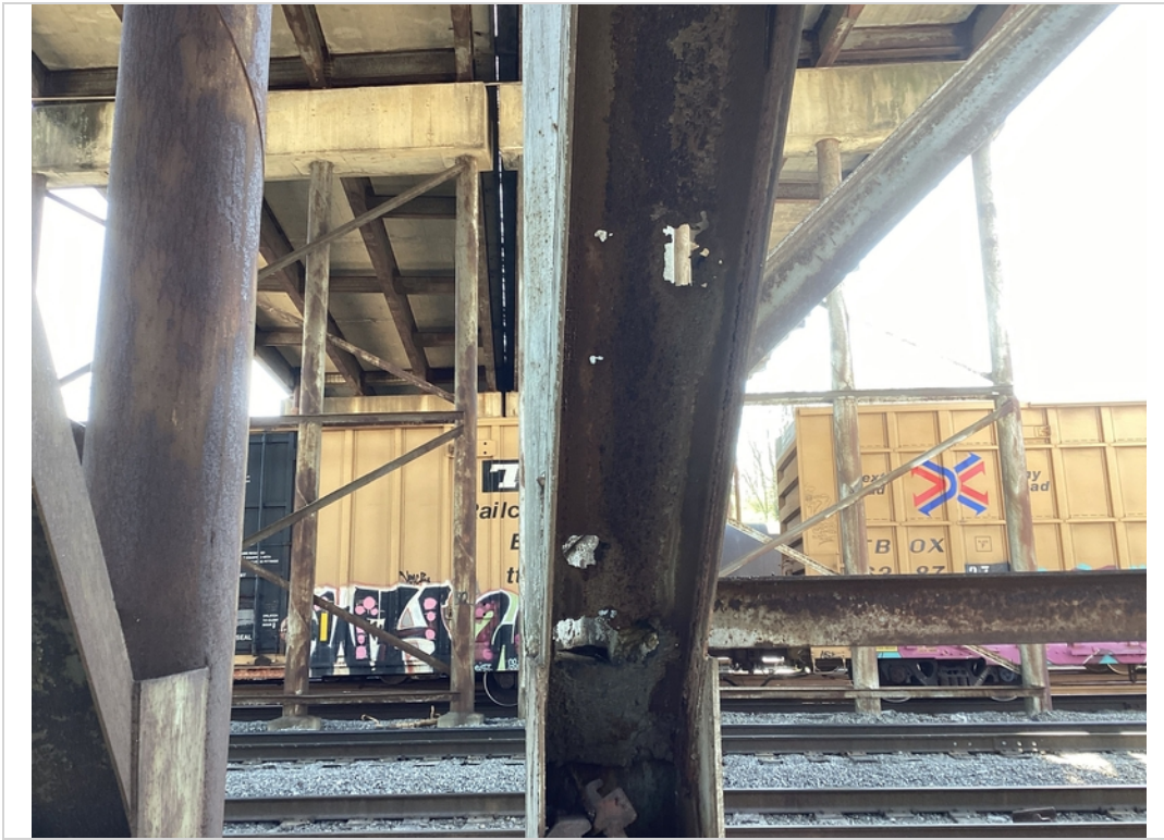
Cross bracing 10-11, diagonal brace, left - multiple holes through
