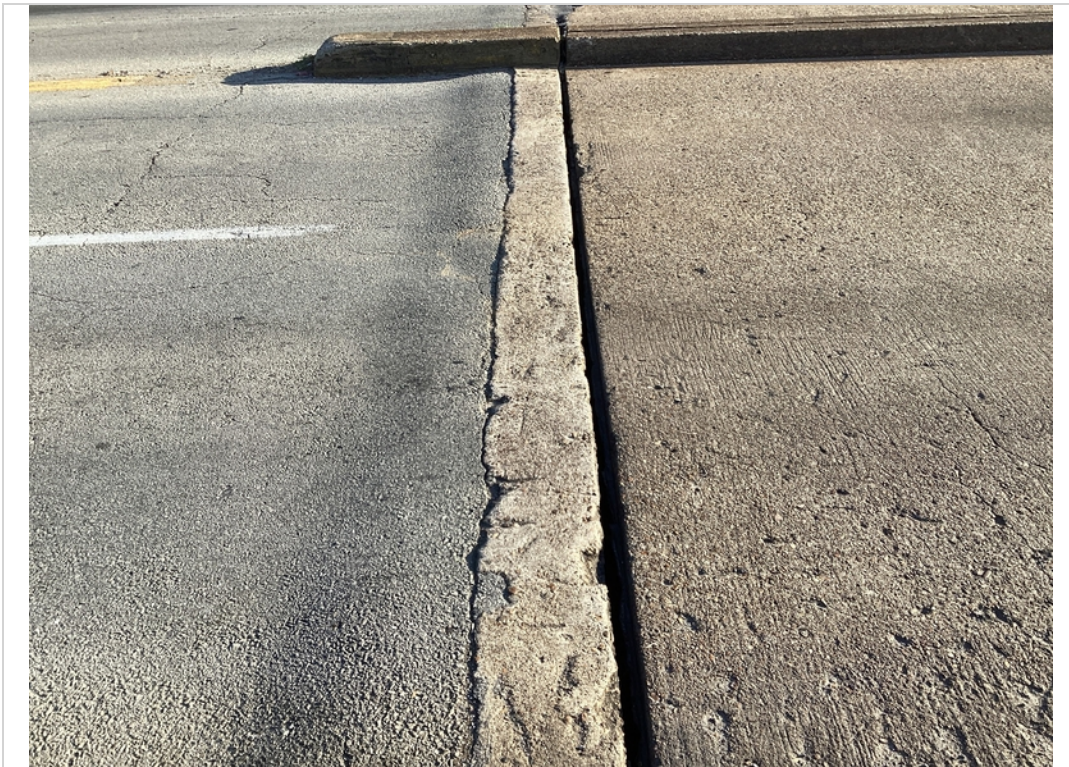
Joint - Approach #1 - Missing Filler
