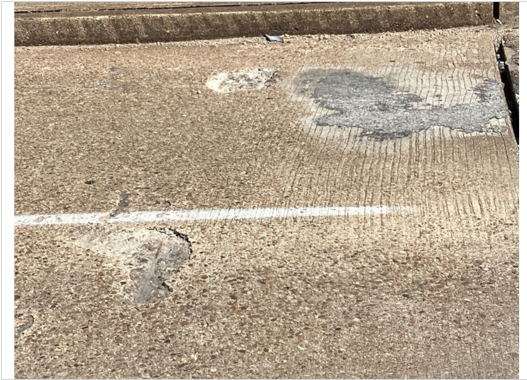
Span 17, wearing surface - potholes, patches
