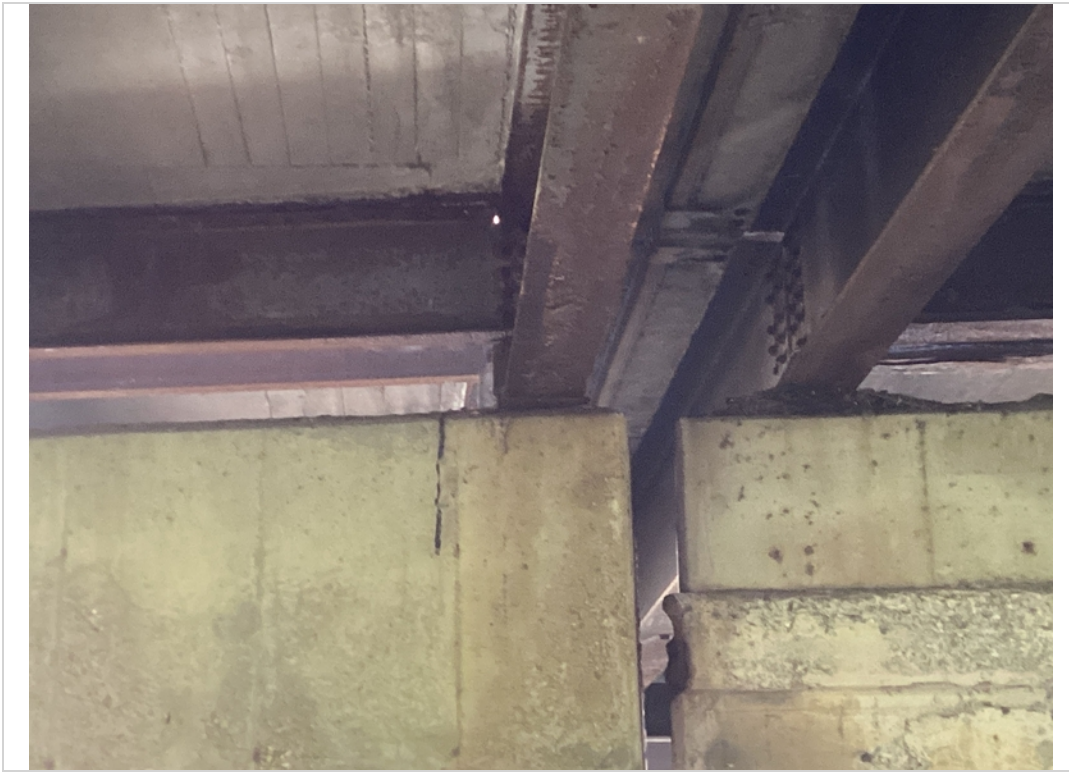
Bent 16, bearing A - missing nuts and bolts on the plate
