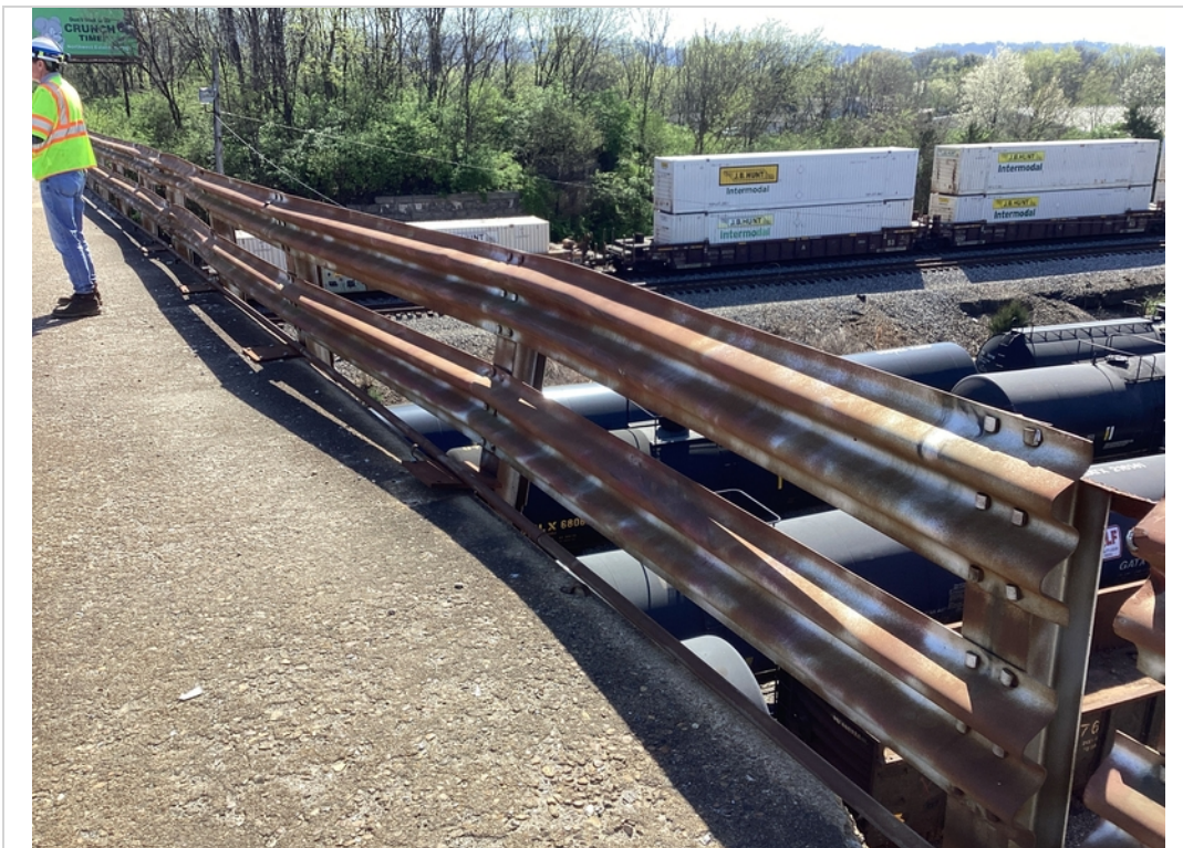
Span 13 - guardrail damage
