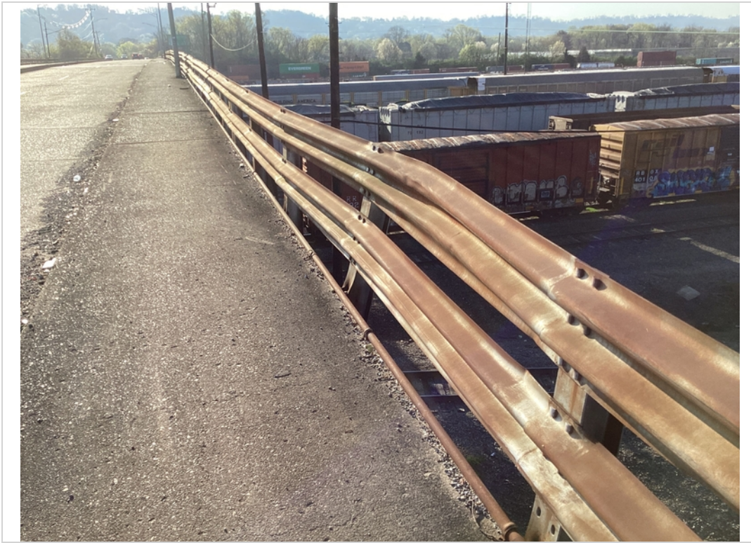
Bridgerail Damage - Span #2 - Right
