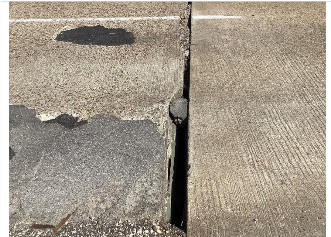
Joint at end of span 11 - rebar spall, breaking up, hole through
