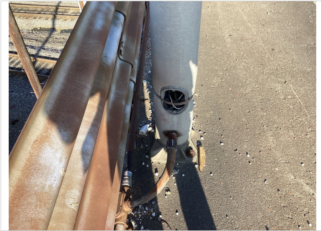
Exposed Wiring - Light Post - Span #4 - Right
