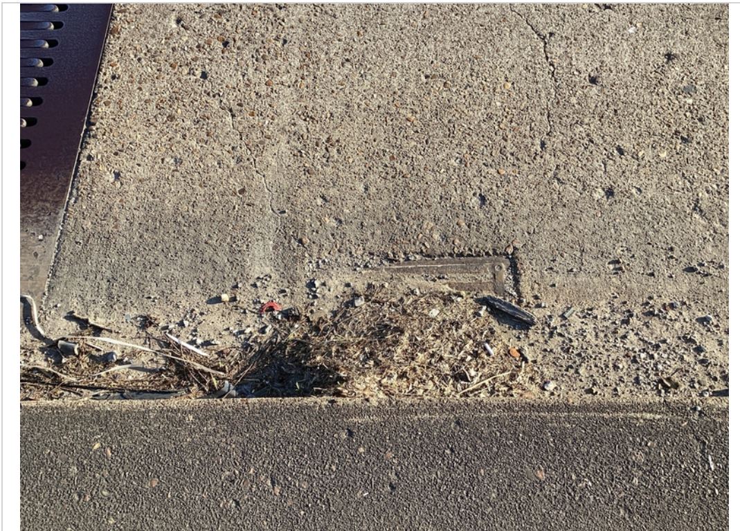
Drain Blocked - Beginning of Span #2
