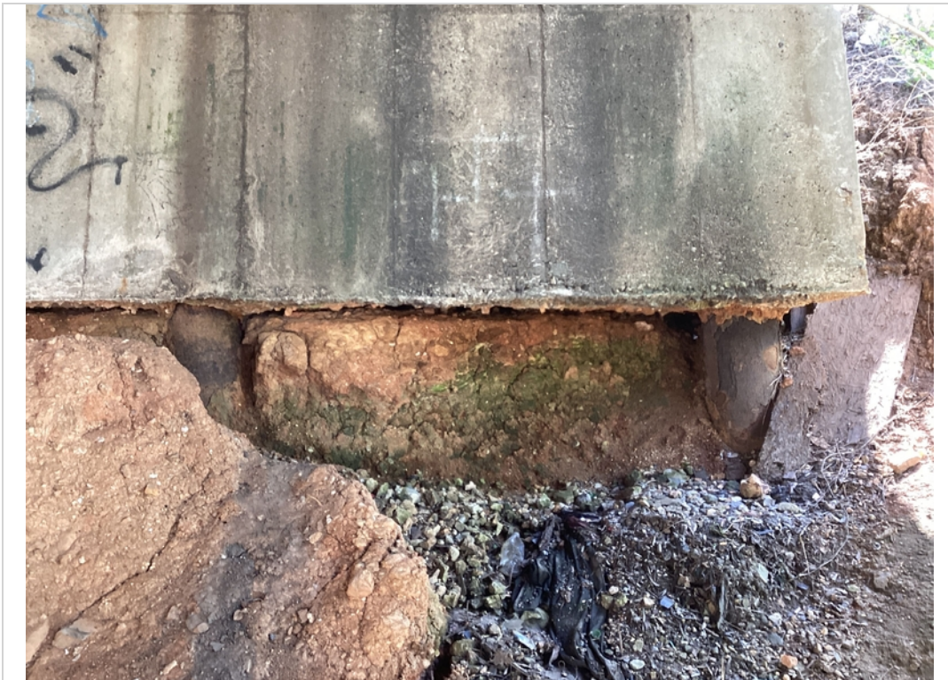
Undercutting and exposed piles with section loss at abutment 2
