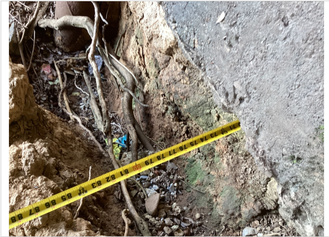
Undermining at abutment 1, right, up to 5' deep
