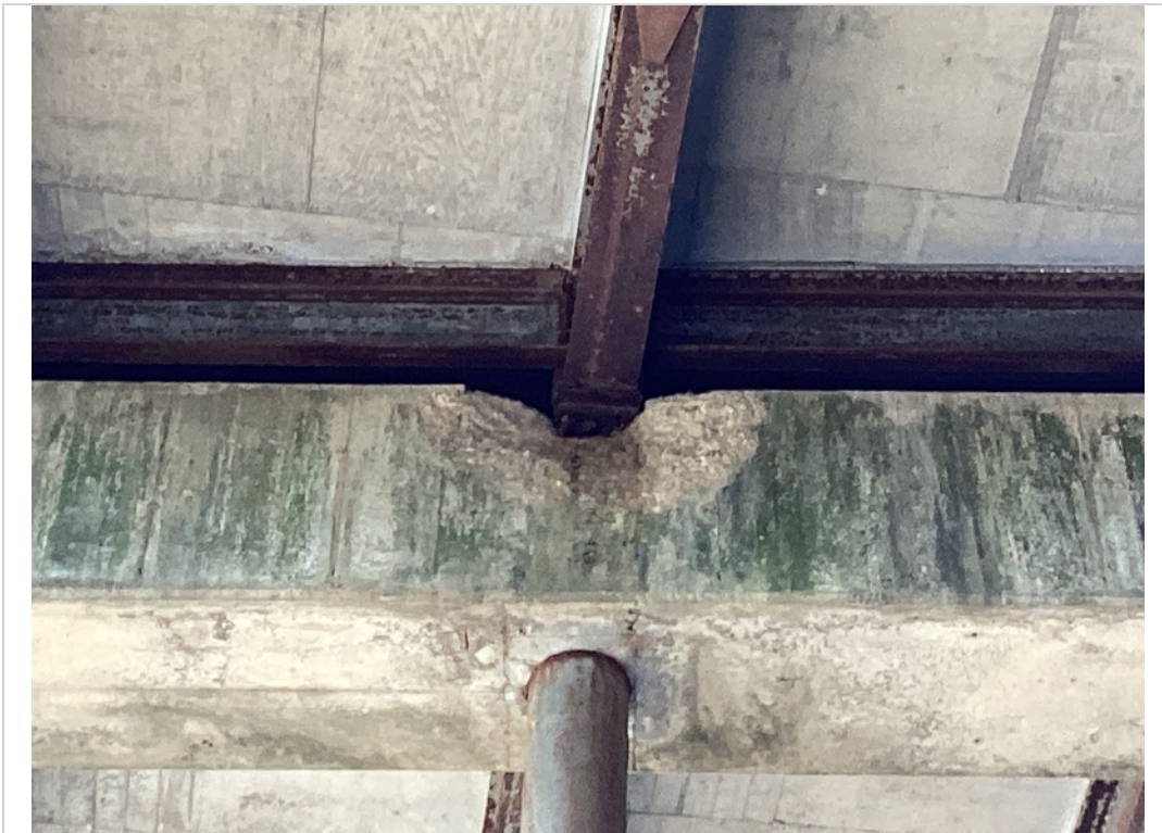
Bent 11, looking back, column B - spalling, loss of bearing area
