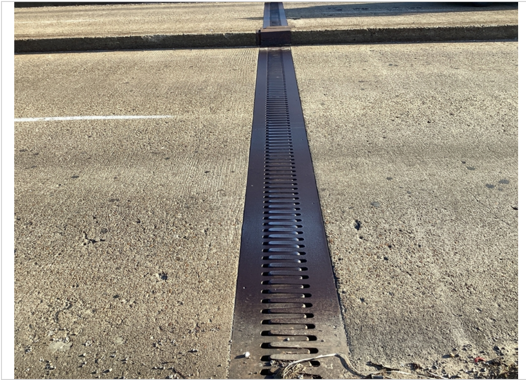
Finger Joint - End of Span #1
