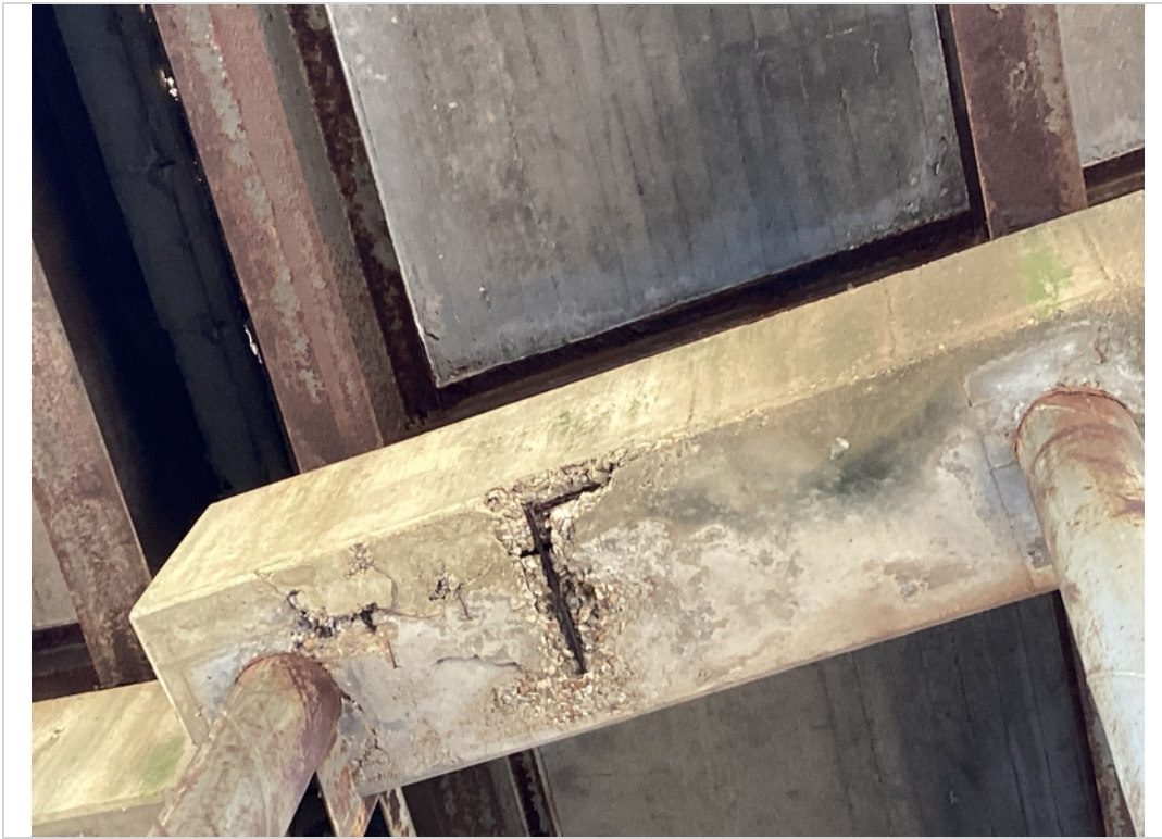
Rebar spall - bent 2, between Beams "A" and "B"
