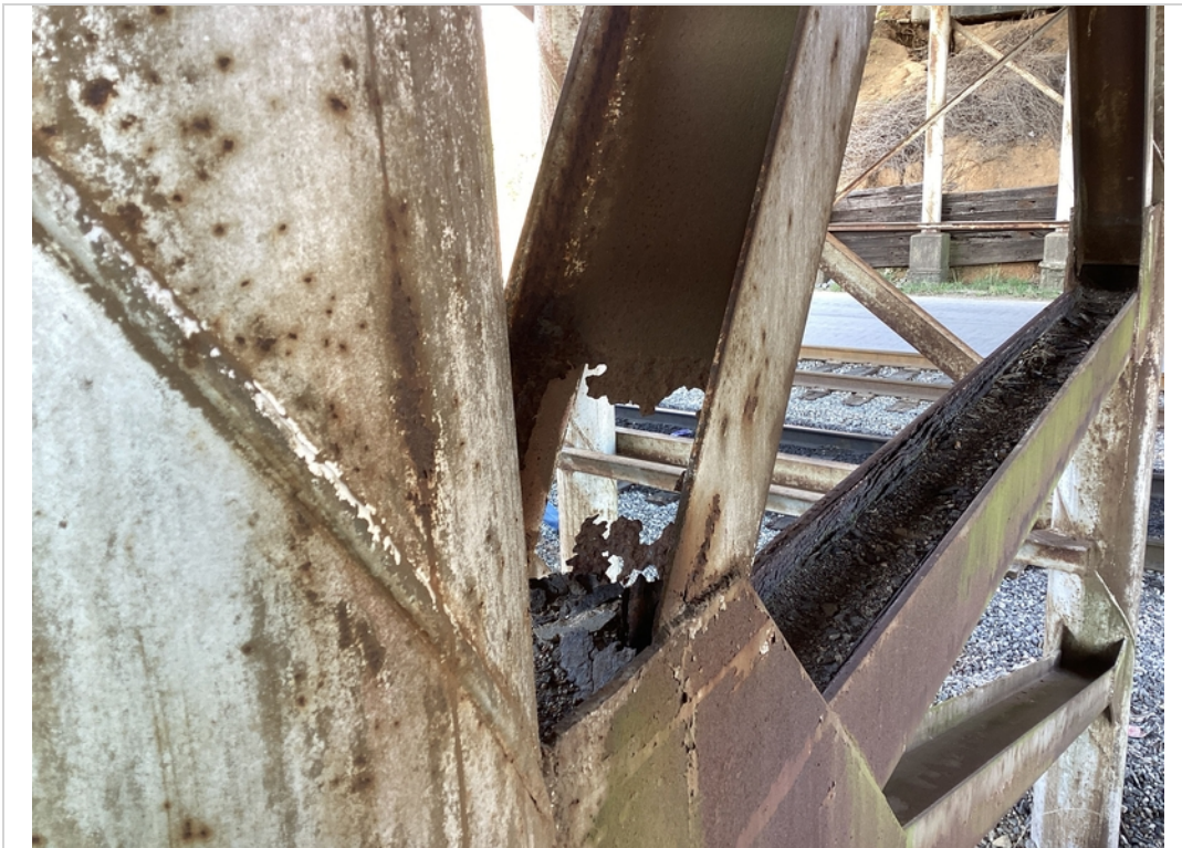
Bent 3, column A - hole through on cross brace, 2-3 left side
