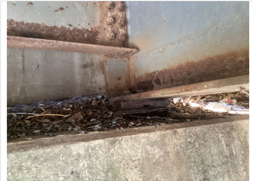
Abutment 1, Bearing "A" - corrosion/section loss
