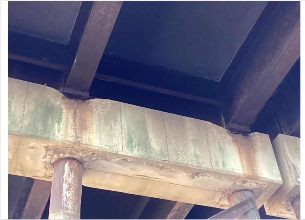
Bent 4, columns A and B, looking back on cap - spalling
