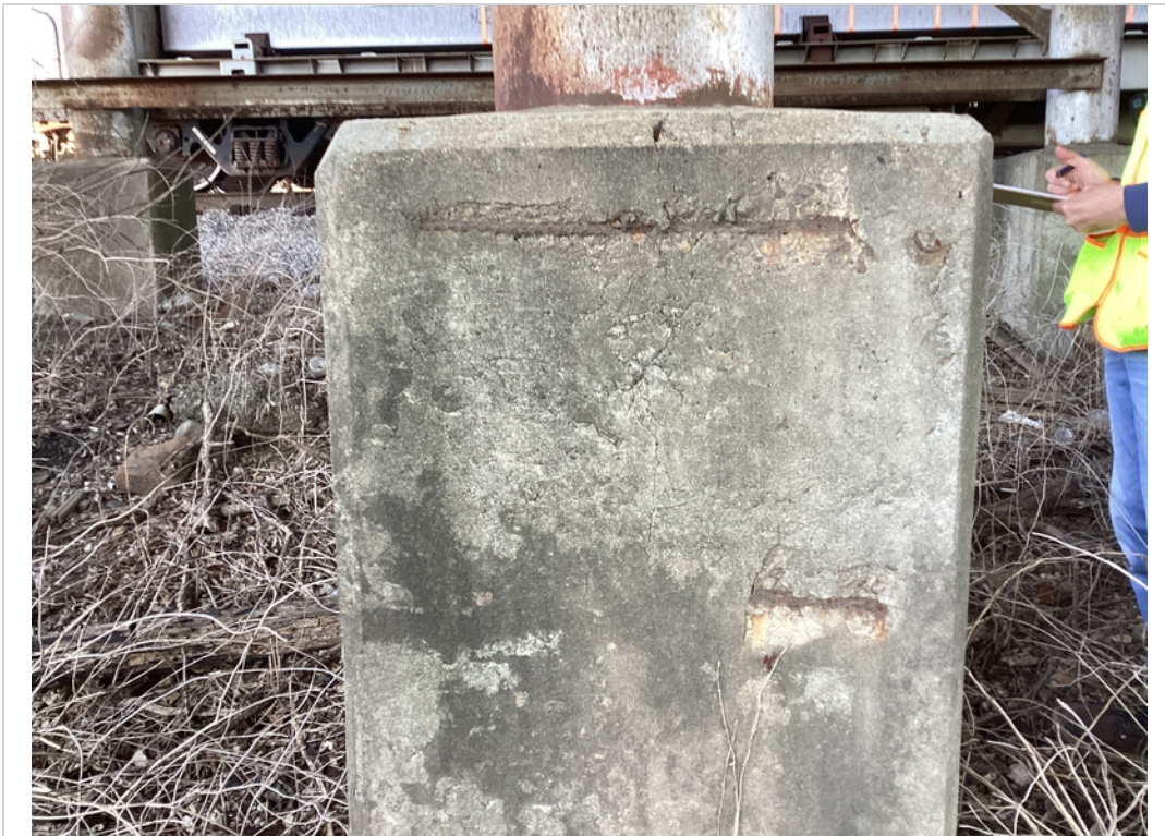
Bent 8, column B, looking back on concrete collar - rebar spalls
