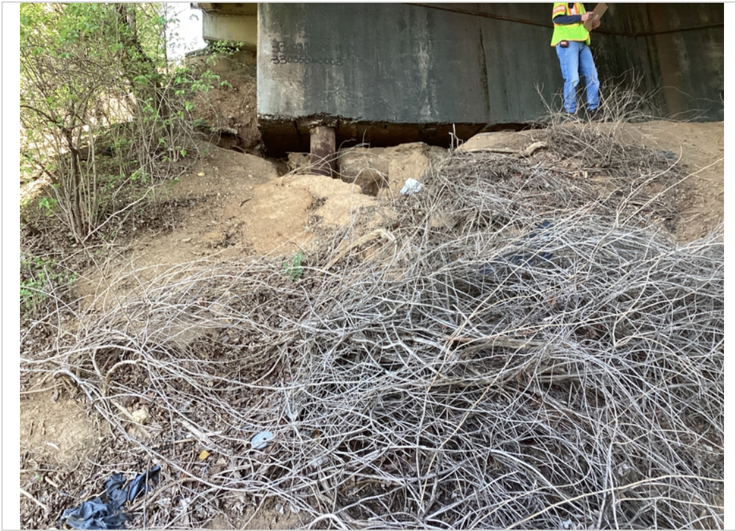
Erosion at abutment 1
