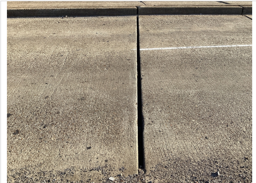
Filler Missing - open Joint - End of Span #2
