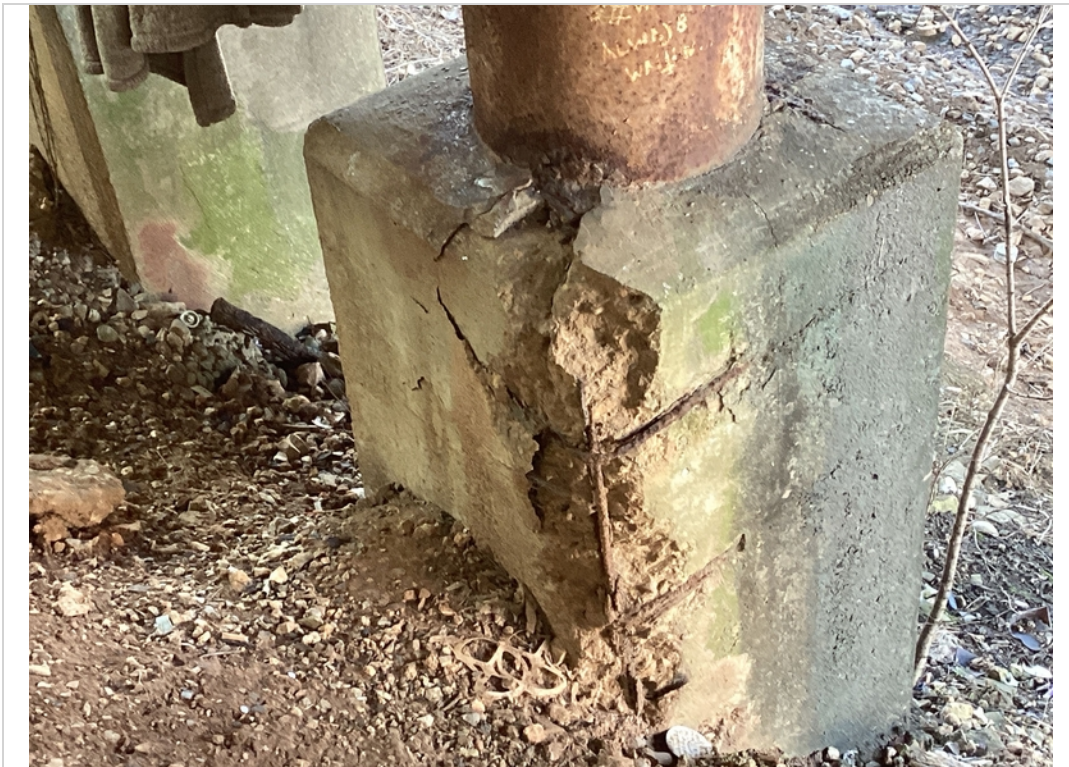
rebar spall - Bent 16, column A, looking back
