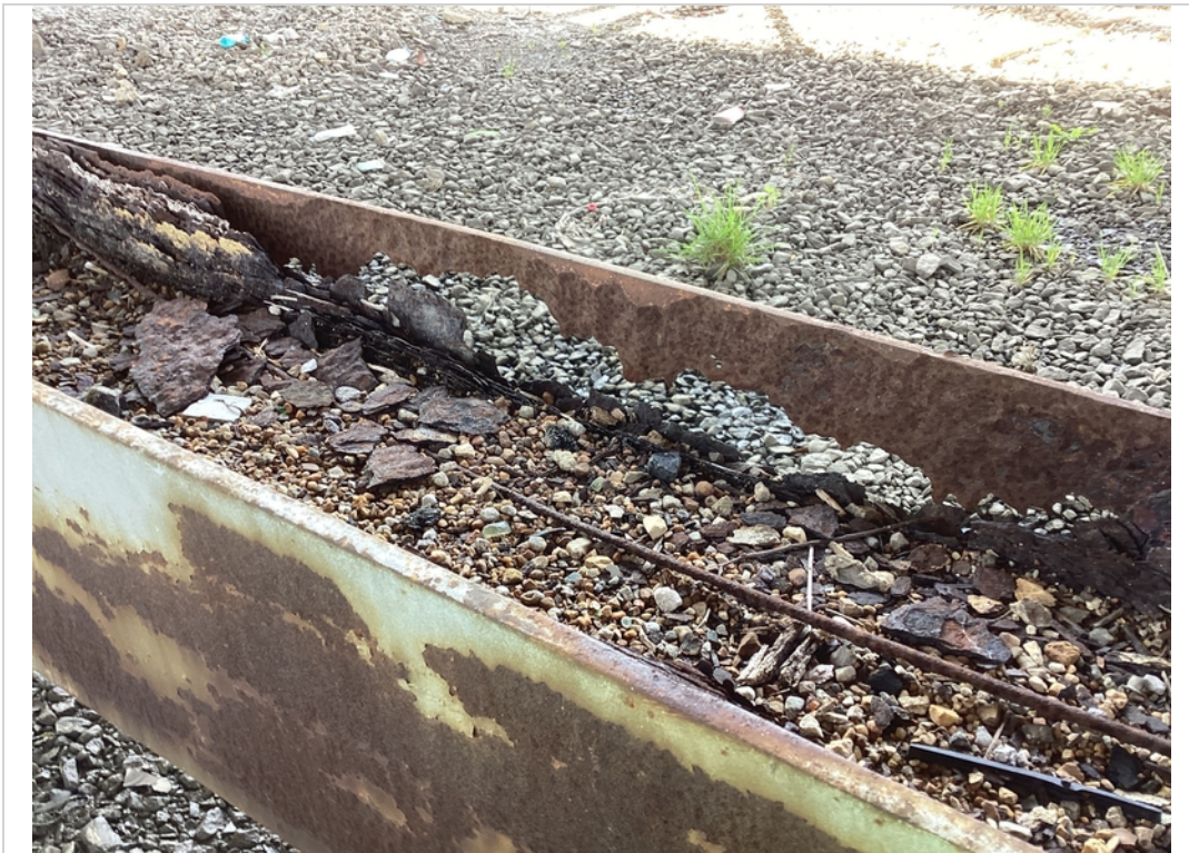
Cross bracing 10-11, left - longitudinal brace has hole through on flange
