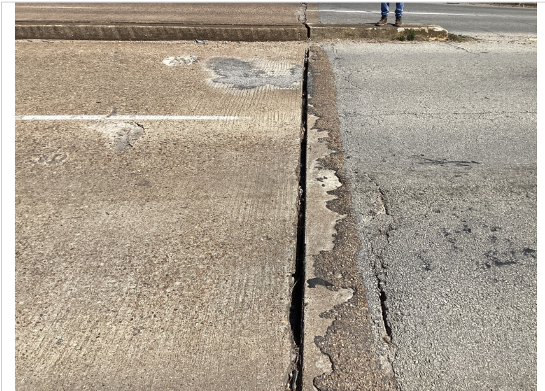
Joint, approach 2 - missing filler
